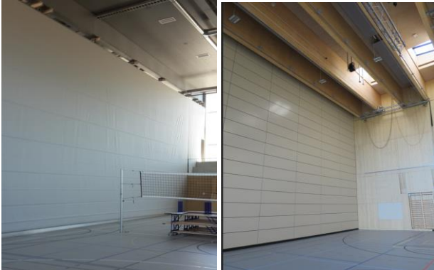
Figure 1. Dividers in sport halls. Left: Curtain. Right: Skyfold acoustic partition
